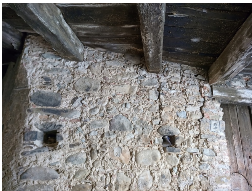
Figura 4 e 5 Interni pre-2022
